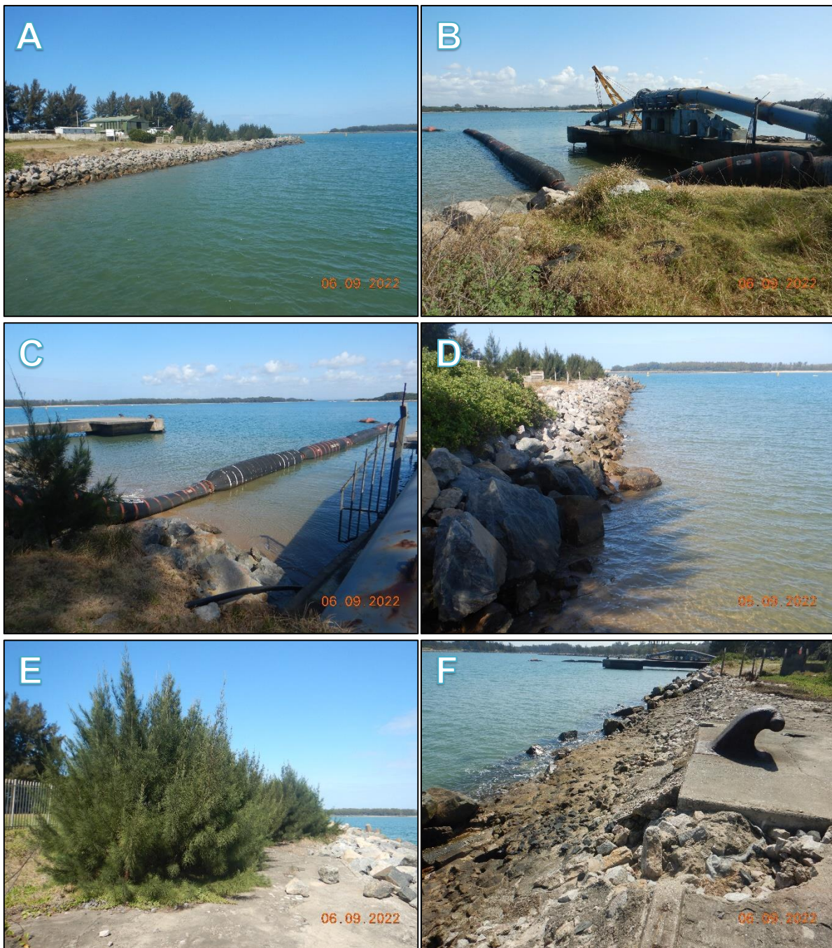
Figure 9: Photographs showing a view of the existing helipad and rock revetment from the estuary (A); T- jetties housing pipelines for pumping of spoil from the dredger (B) and (C); rock revetment along the shoreline (D), Casuarina trees along the line of the rock revetment (E) and a section of the collapsing sea wall that had been covered by rock armouring (F).
